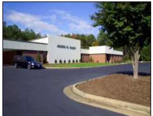
STAPLES MILL 8510 Staples Mill Road Richmond, VA 23228
